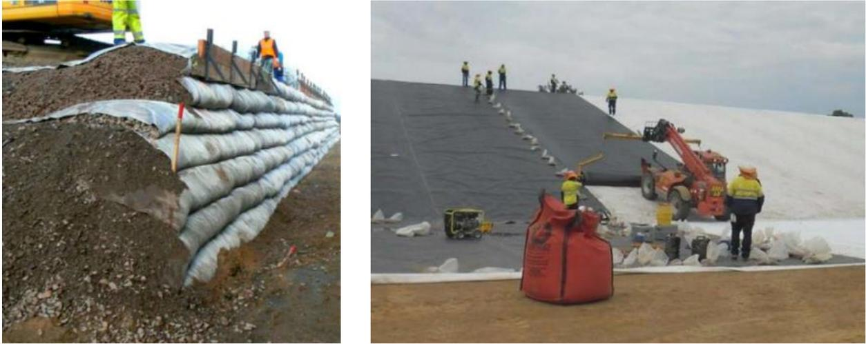
**Figure 3.10: Typical Arrangement of Geotextile Placement / Wrapping**
