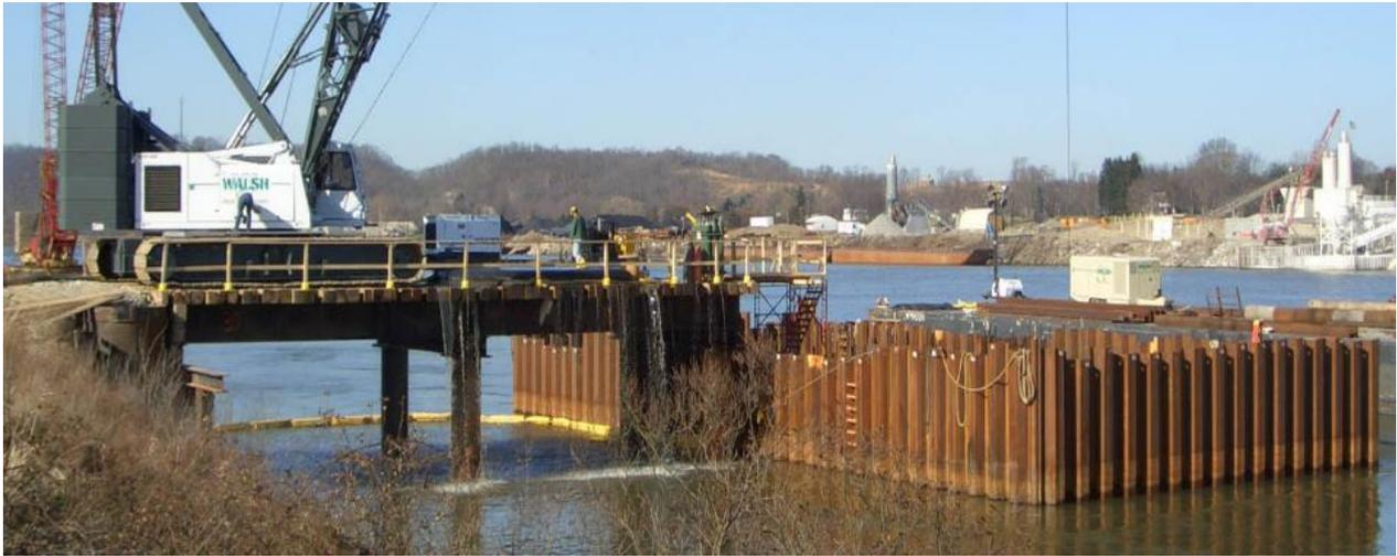
**Figure 3.16: Example of Cofferd Dam**
