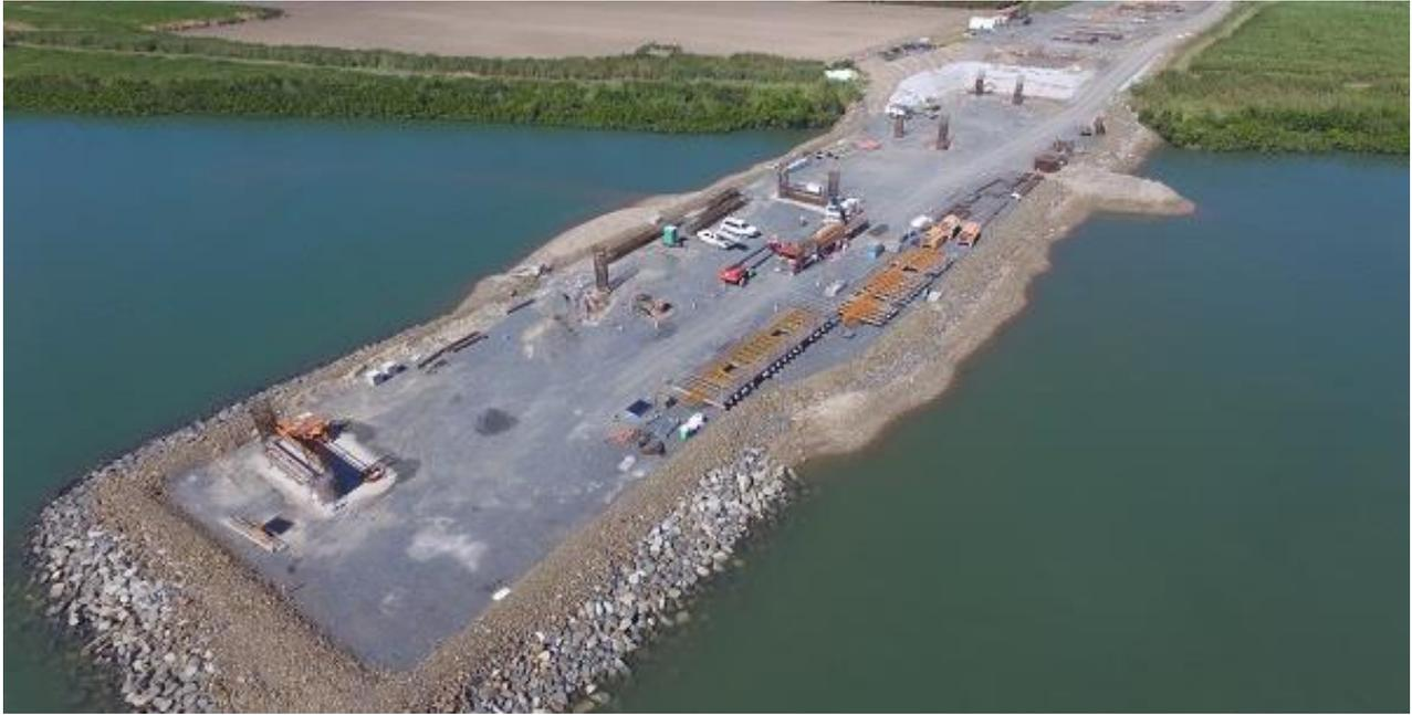
**Figure 3.12: Typical Arrangement of a Bunded Working Platform**
