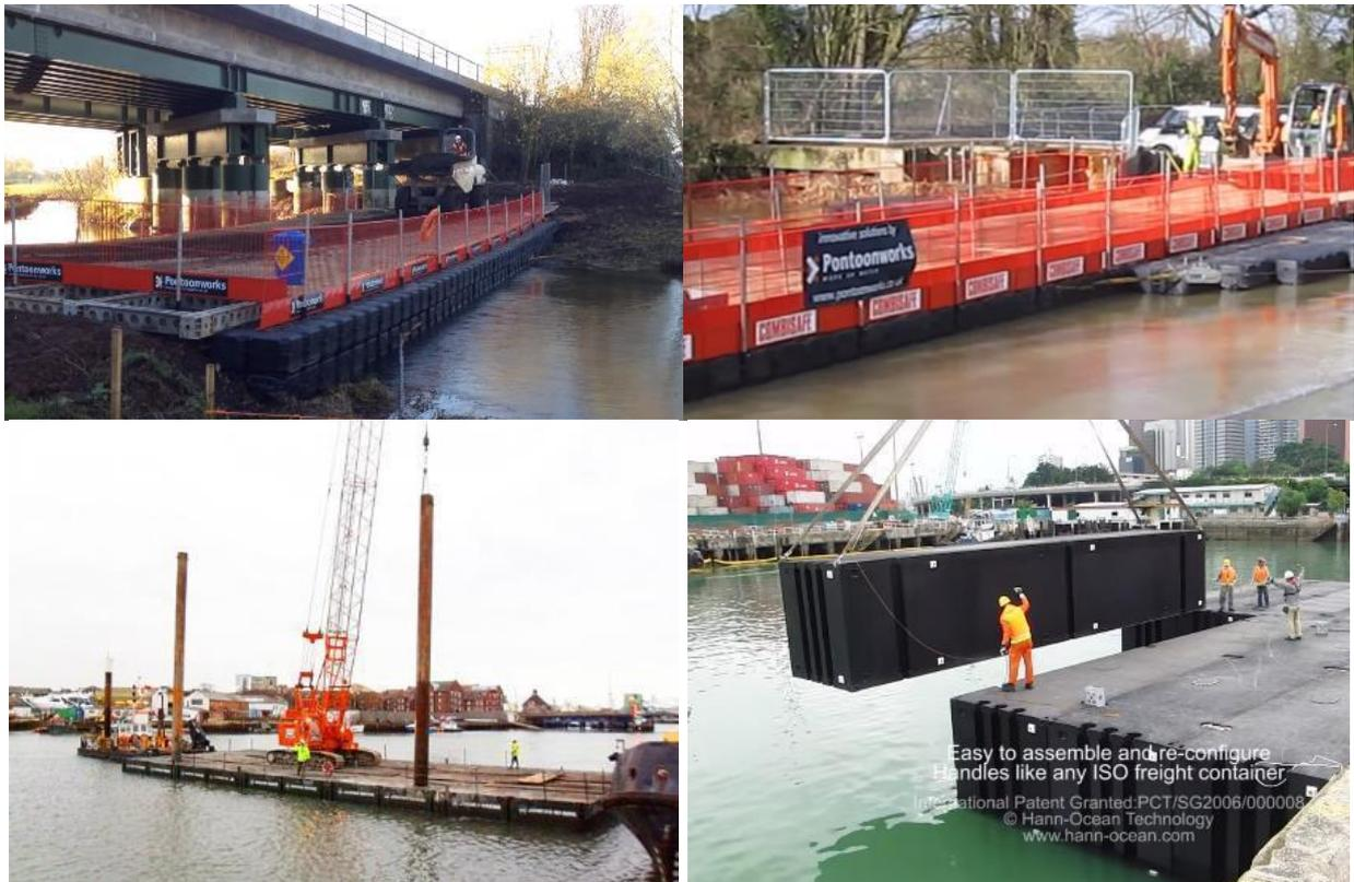
**Figure 3.13: Examples of Modular Pontoons / Floating Causeways / Platform**
