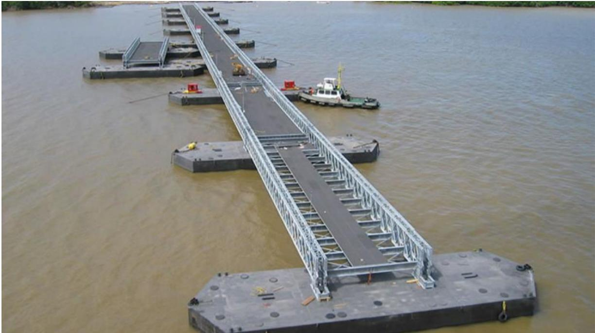
**Figure 3.14: Example of Bailey Bridge with Pontoon Piers**
